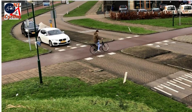
Figure 3.11 - Active travel corridors in Houten, Netherlands
