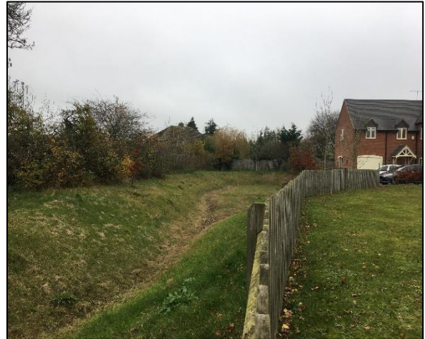
The swale leading to the infiltration basin at Hereburgh Way, Harbury
