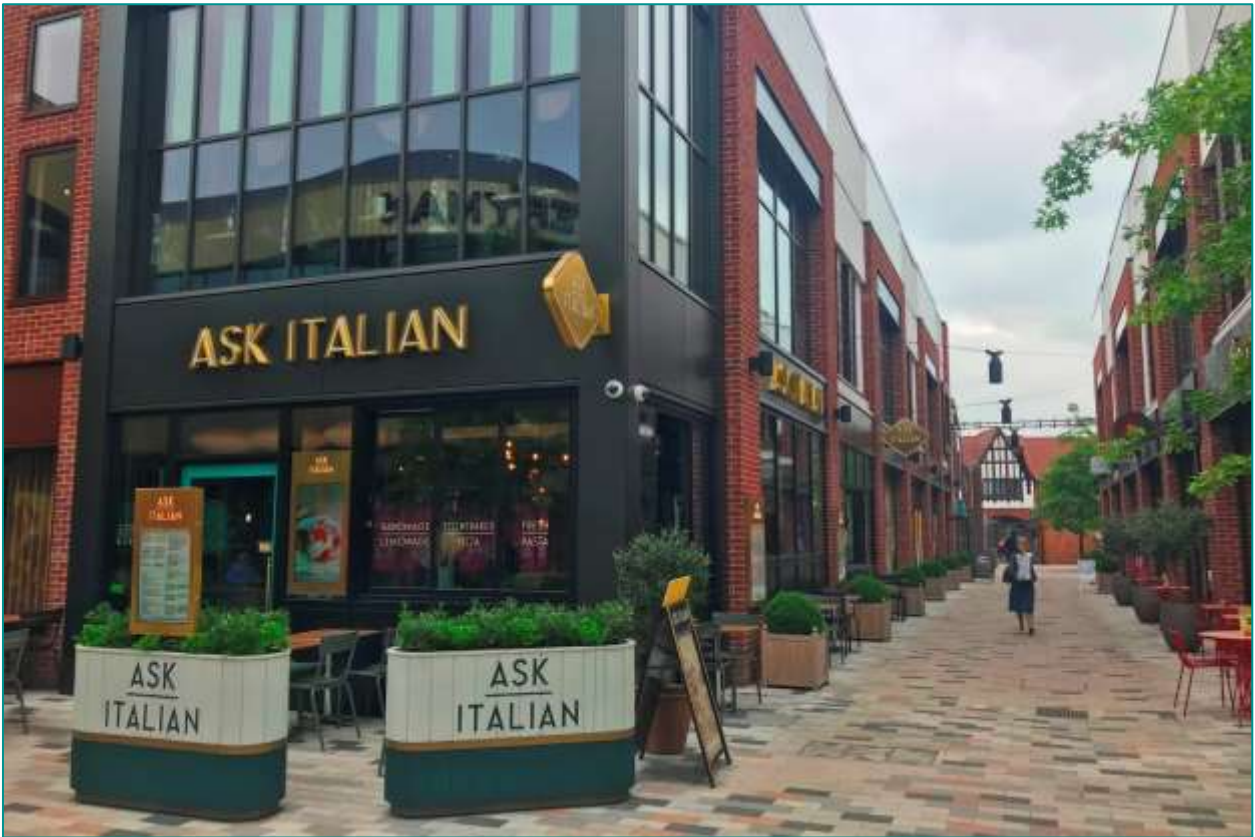
Fig H2. shows a well-designed modern shopfront.
