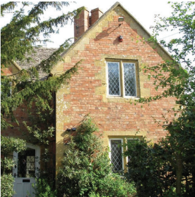
Brickwork at Brookhill Cottage.
