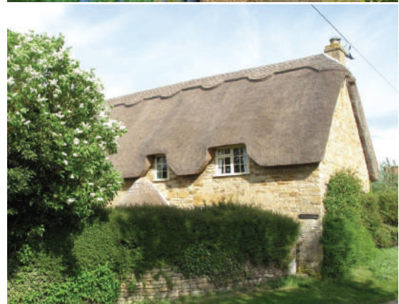
The Retreat – with thatching work in progress (2017).
