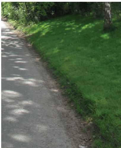
Typical damage to grass verges by passing traffic.
