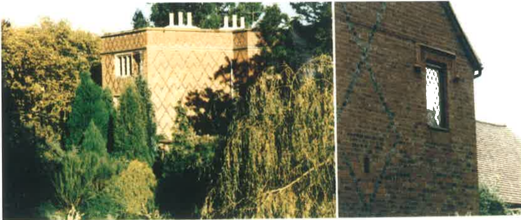
1830's Kitchen Garden House with blue brick herringbone design. 1980's Garden Centre property incorporating herringbone brickwork and window detail
