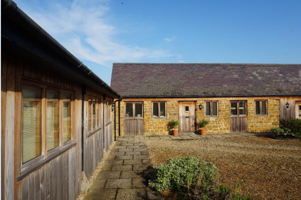
Fig. 19 Manor Farm Business Units
